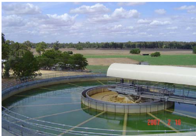
New 50 ML/d clarifier
