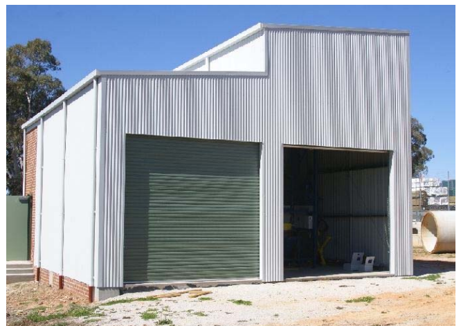
Mudgee PAC System Building
